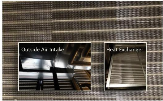
The scope of this project consisted of the replacement of the building's make-up air unit. This unit is responsible for providing fresh air to the building. The age of this equipment, original to the building's construction, pushes it well beyond its useful life. It is inefficient and non-compliant with current environmental codes, The existing equipment was also unable to provide 100% fresh air to the make-up air unit thereby making it operate improperly.
