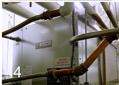
1. Waterproof entire floor of 30th floor mechanical room. 2. New filter system to condition water flowing to residential HVAC units. 3. Relocated a/c units for elevator mechanical room to roof. 4. New air conditioners for compactor and laundry rooms.
