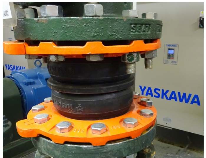
This flexible rubber expansion joint reduces vibration and noise in the HVAC system.
