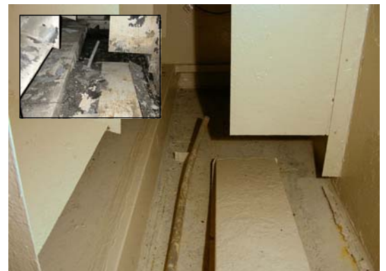
Above left, the exterior of the cooling tower as it appears now with inset photos showing the previous condition. Above right, interior of the cooling tower after repainting with proper paint. Inset photo shows the peeling paint discovered to be the source of the debris in the cooling water system.
