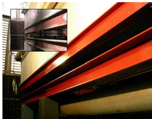
Above left, the exterior of the cooling tower as it appears now with inset photos showing the previous condition. Above right, interior of the cooling tower after repainting with proper paint. Inset photo shows the peeling paint discovered to be the source of the debris in the cooling water system.
