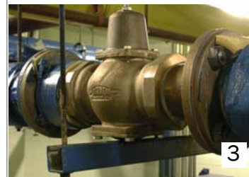
Photographs of some of our completed projects: 1. The KeyTrak system has been installed; 2. The playroom has new carpet; 3. Brass valves have replace corroded carbon steel valves; 4. New digital camera system.
