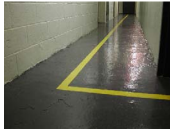
Newly painted with high-gloss paint maing the passageways easier to maintain.
