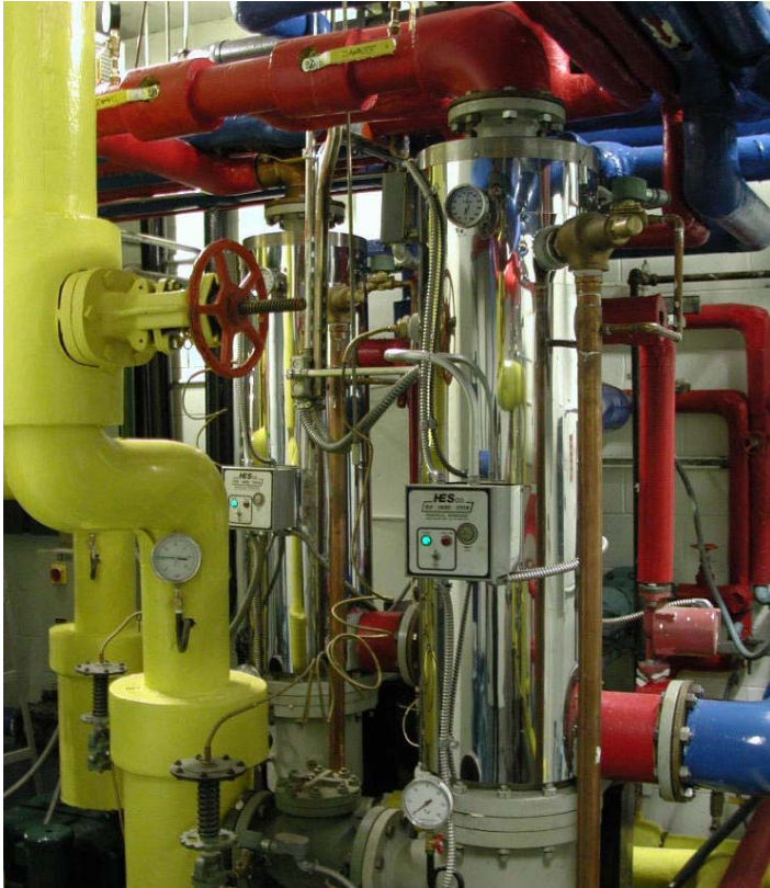
Two of the four new stainless steel water heaters now installed. These units are more
