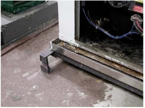
The original installation made it impossible to drain the system (top), the new installation places the unit in a pan that can be drained easily (above).
