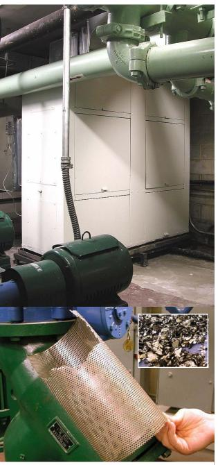
This screen in one of the main water circulation systems for the HVAC system was found to be broken. Inset shows debris that had accumulated in screen.
