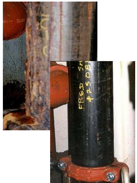
Above left you see the standing water and mold indicating serious long-term neglect. The water leaks were caused by badly maintained valves. Above right you see the clean and dry floor now that the valves have been repacked. This is basic but important maintenance.
