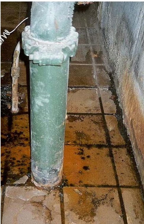
Above left you see the standing water and mold indicating serious long-term neglect. The water leaks were caused by badly maintained valves. Above right you see the clean and dry floor now that the valves have been repacked. This is basic but important maintenance.
