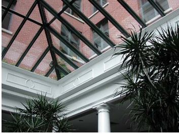
Newly painted and re-planted atrium.
